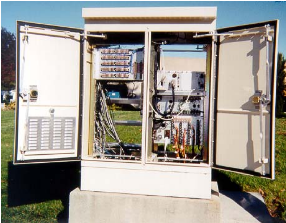
Figure 3 - Type 333 (dual rack) Cabinet with Additional Detector Panel
