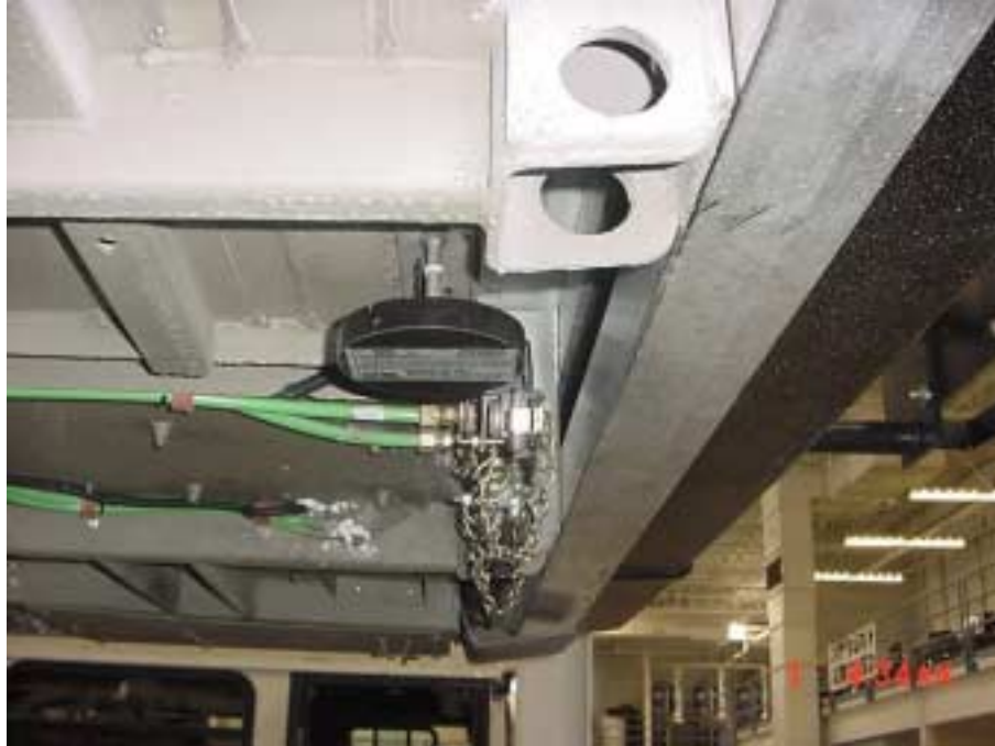
Figure 6 Transponder mounted on underside of bus
